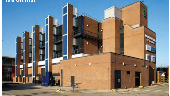
The microgrid at the Energy Centre is a UK first
